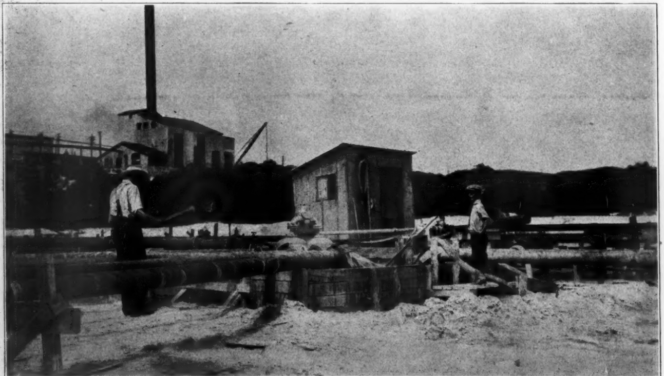
Sump Where Lines From Pulsometers at the Different Mining Operations Converge and Discharge into a Common Sump
